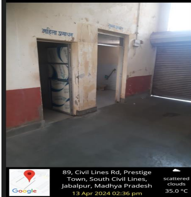
Figure 2a : Disabled Friendly Washrooms
